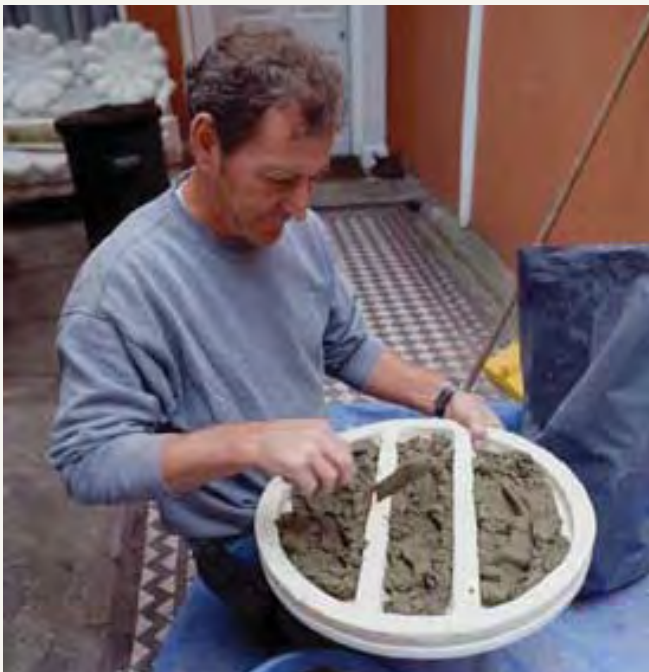
67 Installation of the plaque to Madame Marie Tussaud (1761-1850) at 24 Wellington Road, St John's Wood, London, in 2001. The ceramic plaques erected by English Heritage are about 2 inches (51 mm) thick, and their backs are partially hollowed out to reduce weight.
