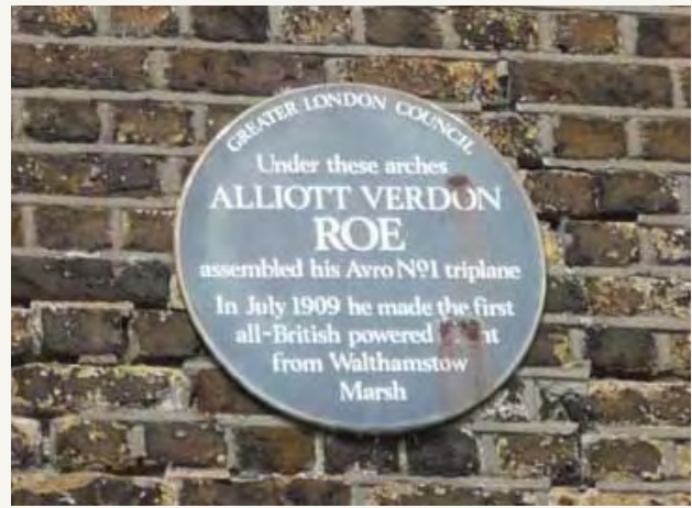
82 This GLC plaque of enamelled steel was erected on a railway viaduct in Walthamstow Marshes, London, commemorating a site associated with the aircraft designer and manufacturer A.V. Roe (1877-1958). Put up in 1983, it was in poor condition 20 years later, reflecting both exposure to the elements and vandalism.
