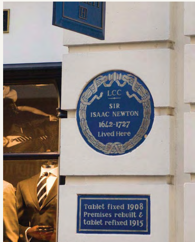
85 Where a plaque marks the site of a building, or is re-erected on such a site, it will be important to make this fact clear. For the short time that this practice was followed under the London-wide scheme, old plaques were re-erected along with supplementary tablets; an instance is this plaque commemorating Sir Isaac Newton's residence in Jermyn Street, St James's.
