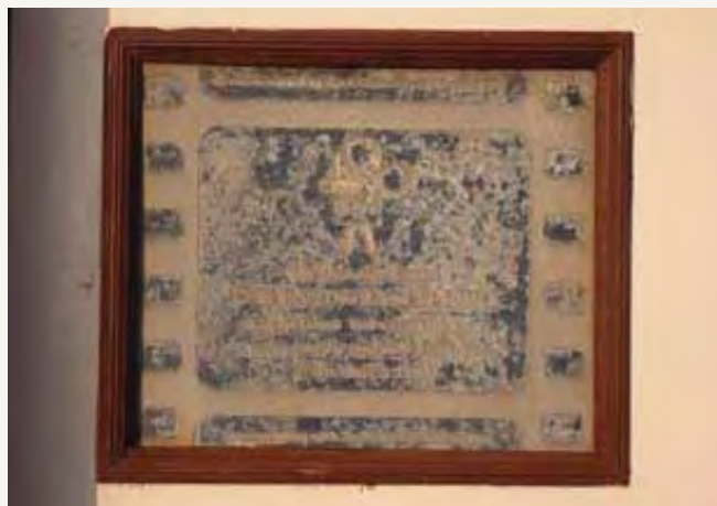
44 Certain atmospheric conditions can be detrimental to plaques, especially those made of metal. This is well illustrated by the plaque erected at 132 Kings Road, on Brighton seafront, by Cinema 100, in association with the British Film Institute. It marks the site where, in 1896, films were first shown to the public outside of London.
