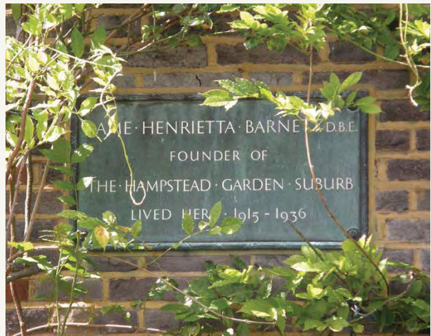
80 The growth of climbing plants, trees and shrubs can damage a plaque, and can inhibit visibility. Here, wisteria has begun to cover the plaque to Dame Henrietta Barnett (1851-1936) at 1 South Square, Hampstead Garden Suburb, London.
