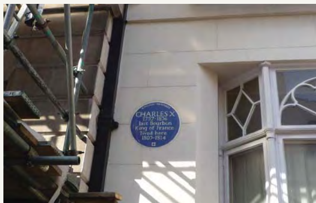
79 Wherever possible, plaques should be protected while building and decorative works are carried out. Shown here is the English Heritage plaque to Charles X (1757-1836), last Bourbon King of France, at 72 South Audley Street, Mayfair, London.
