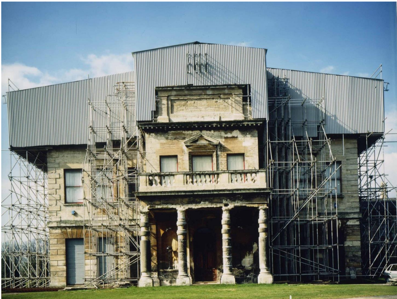
Fig. 4. Exterior conservation in progress. © English Heritage
