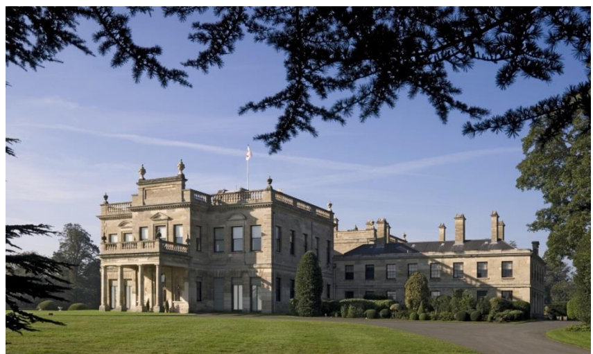
Fig. 1. Brodsworth Hall, Yorkshire. © English Heritage.
